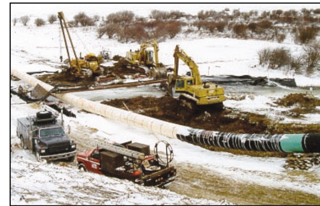
A work in progress. To reduce time in-stream, a temporary bridge was placed across the creek and the pipe is prepared ahead of time. The creek water is being pumped around the work station and discharged downstream.
