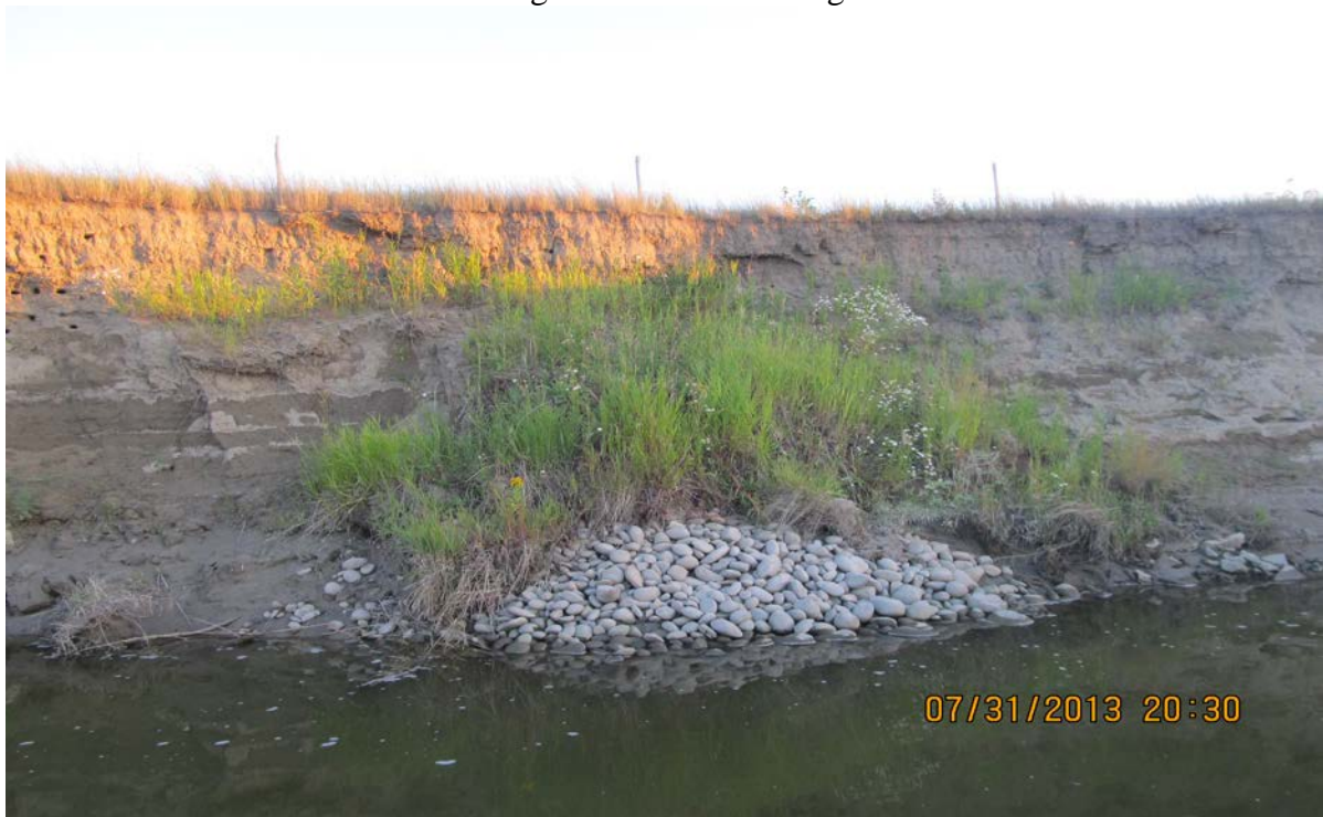
Photo 10 – Photo showing active lateral cutting and rip rap that was brought in.
